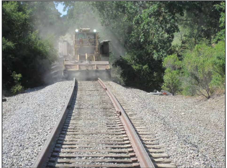
Ballast regulator brooming the track.
