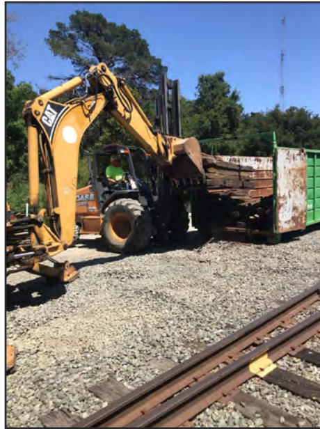
Stephen Barkkarie photograph Chris Campi runs forklift to load ties.
