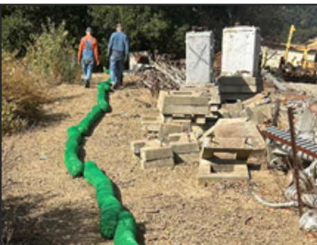
SiltSoxx erosion-control booms. John Link & Ron Thomas in distance.
